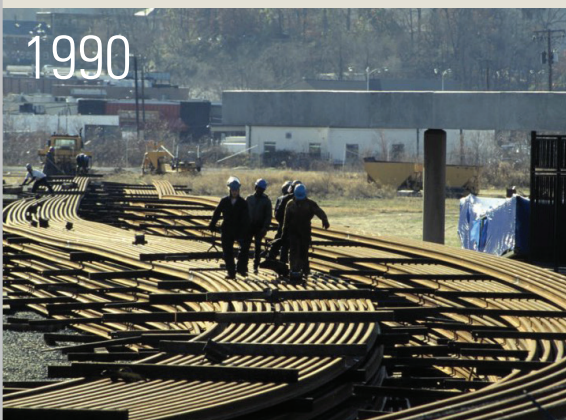
Construction workers walk along the massive strands of rail that will be welded and installed along the Green Line at West Hyattsville.
